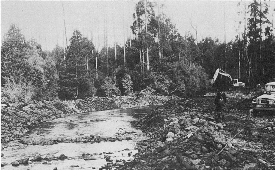
Reconstruction work at Mountain Creek, Lake Sorell.
