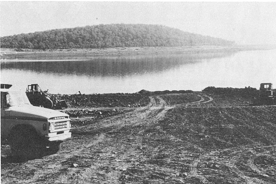
Boat launching ramp under construction at Swan Bay, Great Lake.
